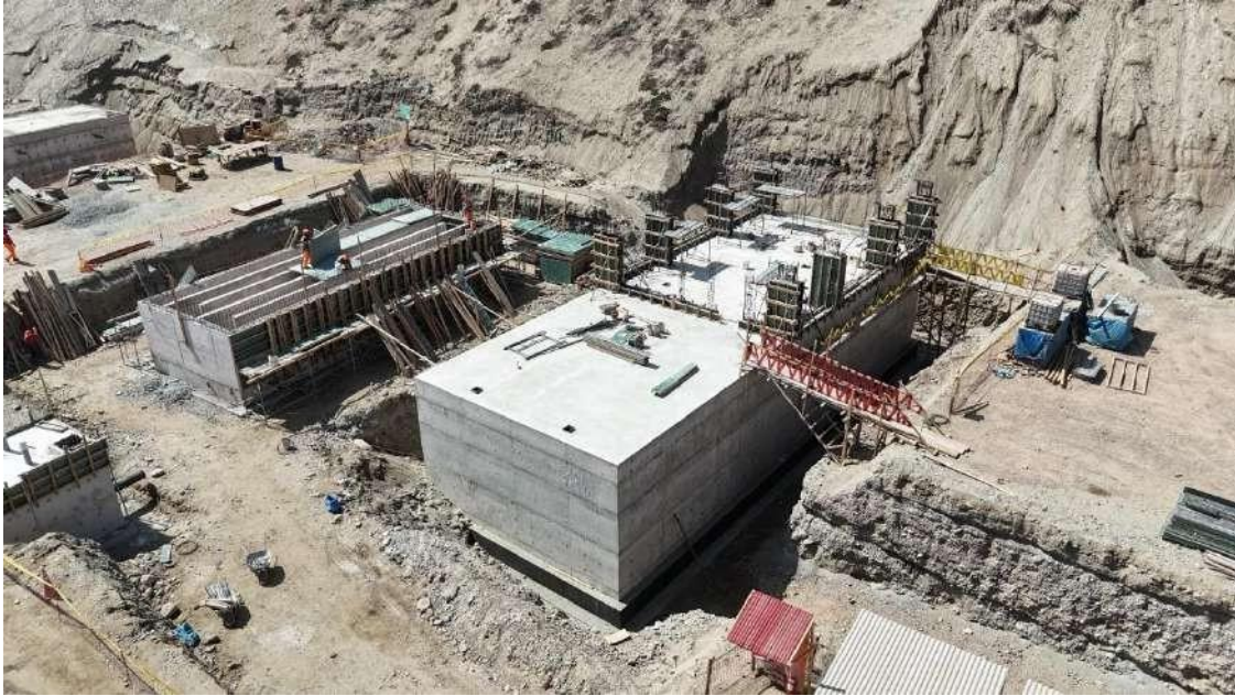
Aerial view of progress at the Drinking Water Treatment Plant – 32% progress
