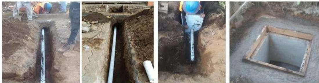
Installation of manholes
