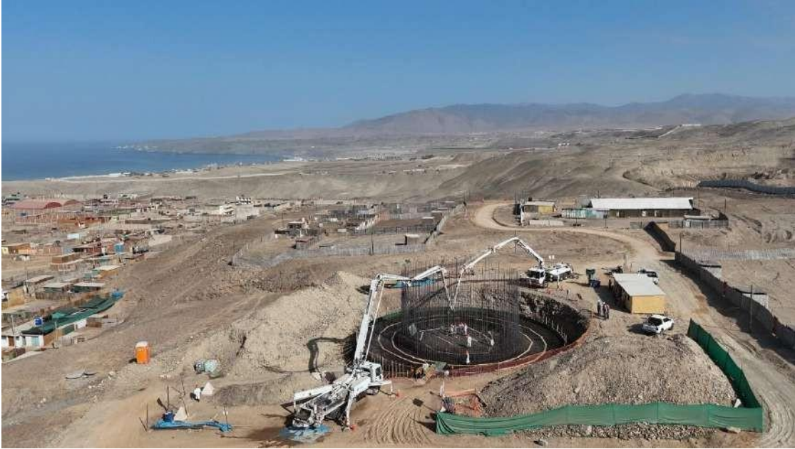
Concrete placement in REP-01 elevated reservoir, 2000 m 3
