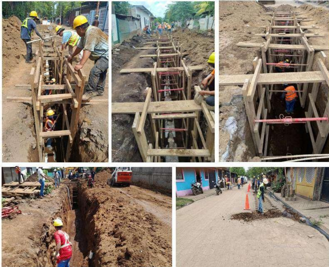
Installation of sanitary piping
