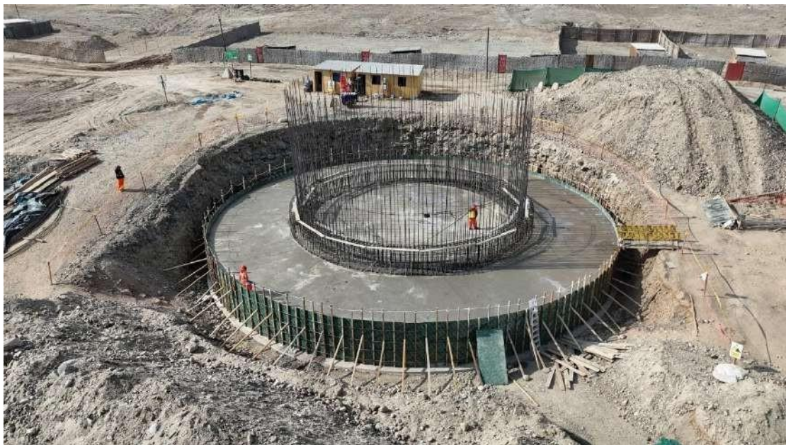
Completion of pouring into elevated reservoir REP-01, 2000m 3
