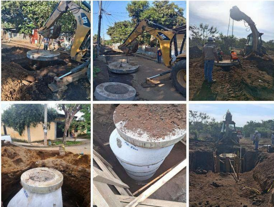
Installation of manholes
