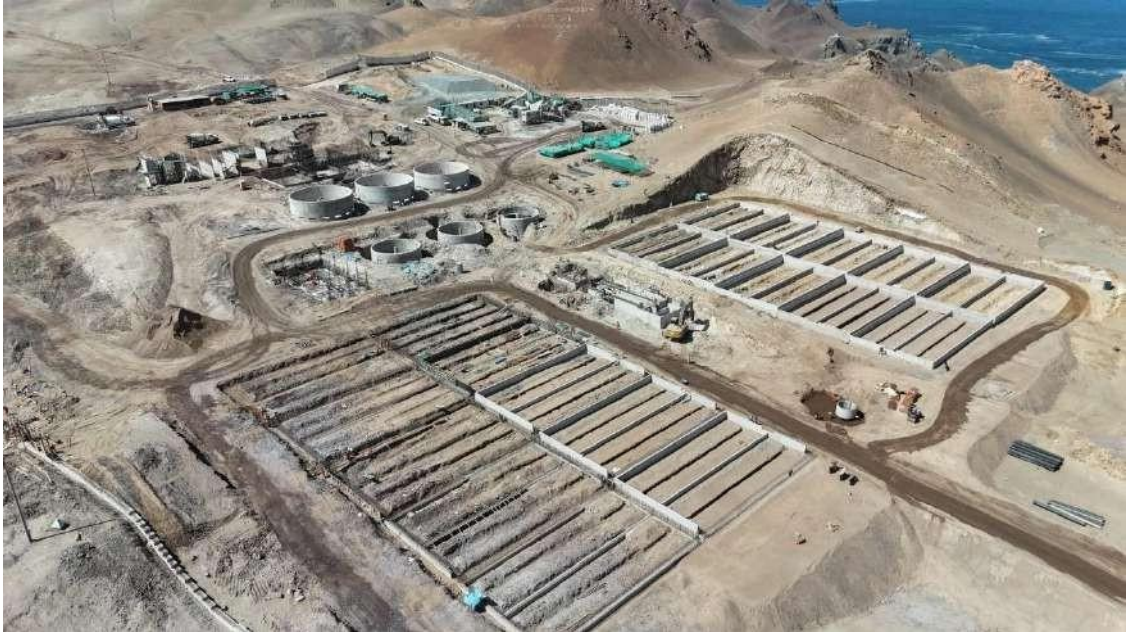
Aerial view of the PTAR – Chala Wastewater Treatment Plant
